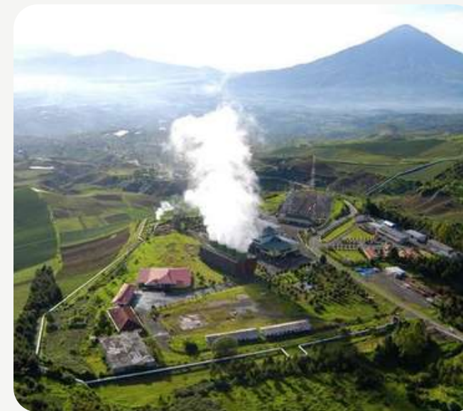
Pictured: Darajat Geothermal, Indonesia. One of the many projects being supported by this initiative.
